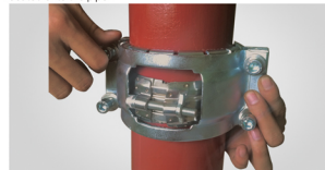
3、將螺絲橫向擰緊，使兩側板的平行間距相同。Tighten the screw crosswise alternatively so that the two plates are put in parallel with the same spacing.
