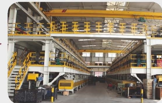
End Grinding Line
